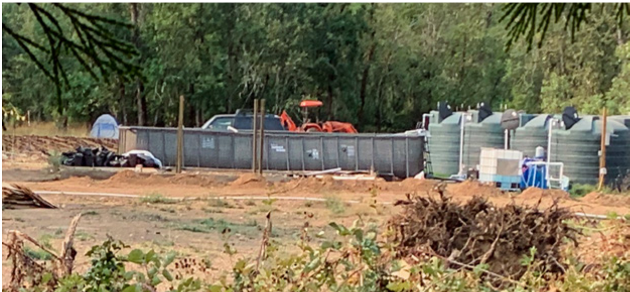
Photo courtesy of an anonymous community member -- water tanks and fertilizer pool -- 2021
