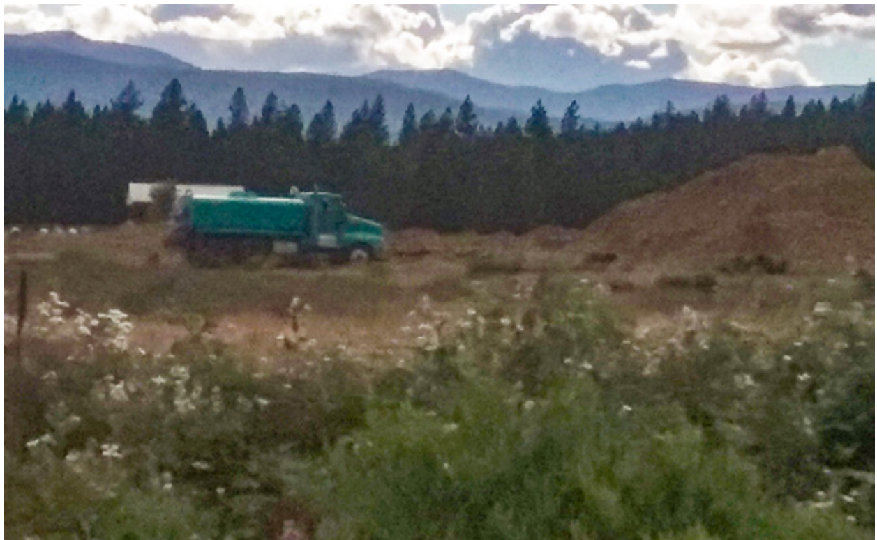
Water truck filling up at an unpermitted acre-foot sized hole -- 2021
